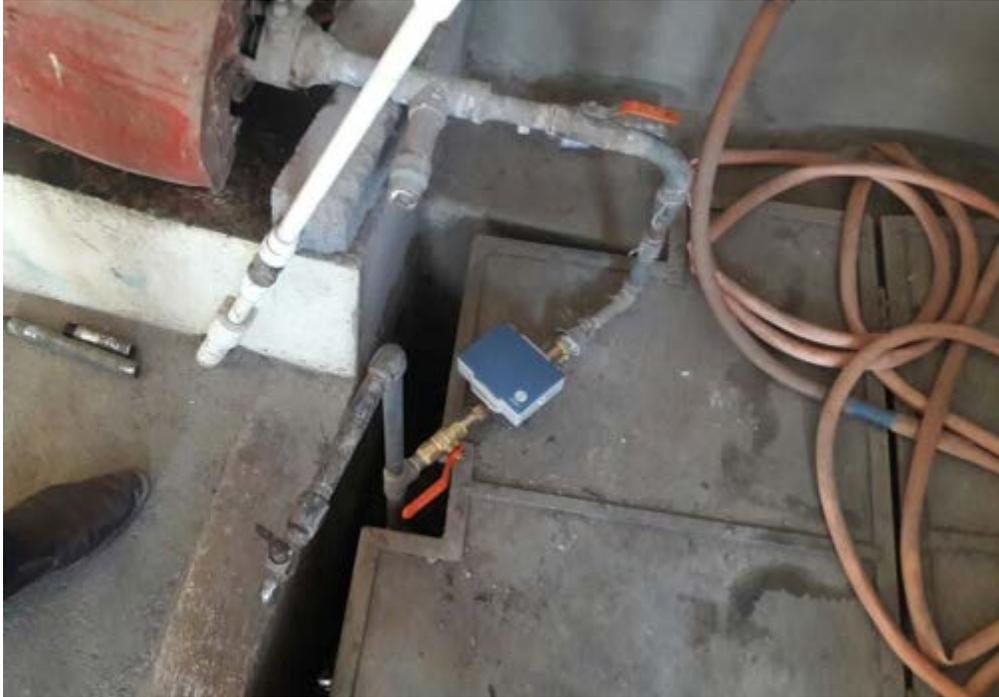
Figure 7: Water meter pipe installation
