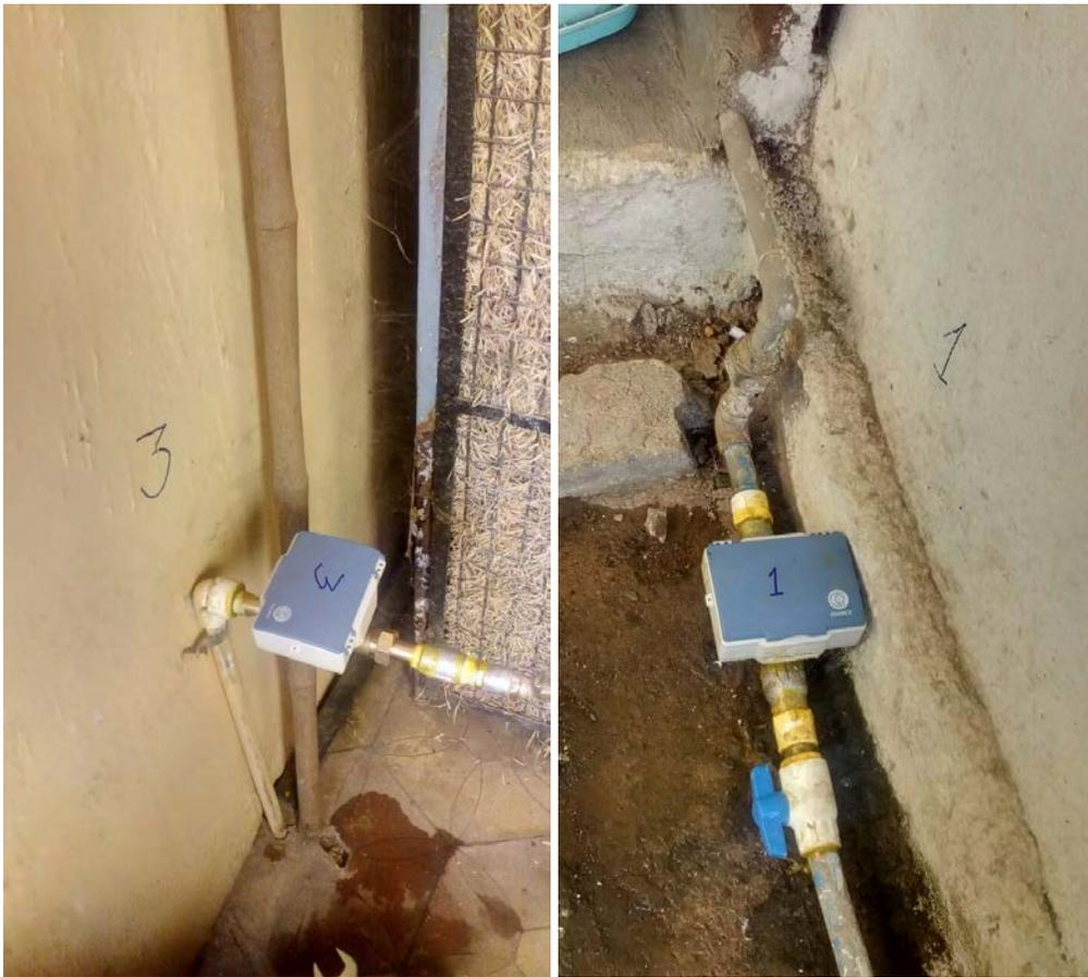
Figure 8: Water meter pipe installation
